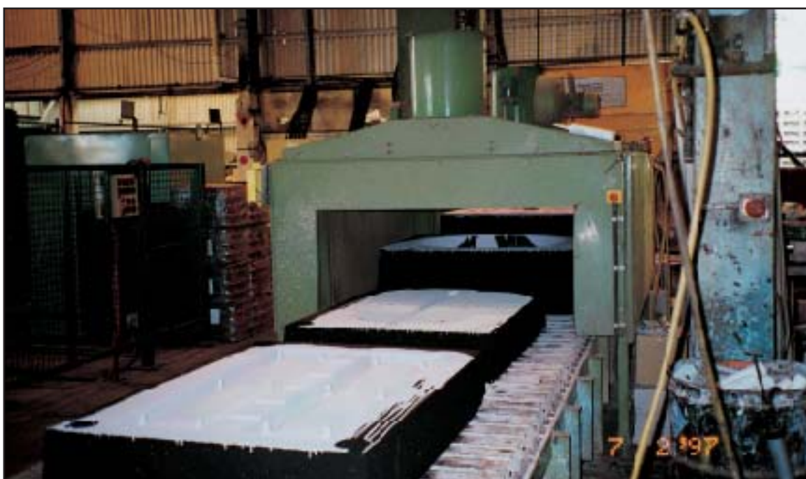
● Infrared drying tunnel for mould wash
