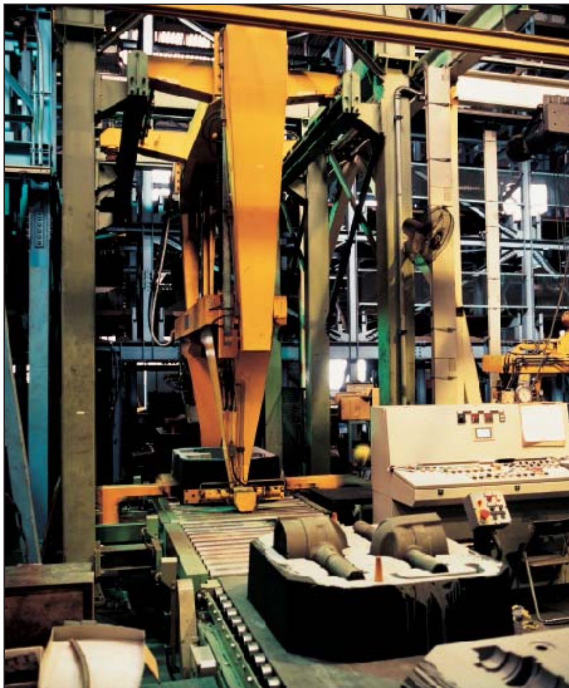
View of automatic closure
